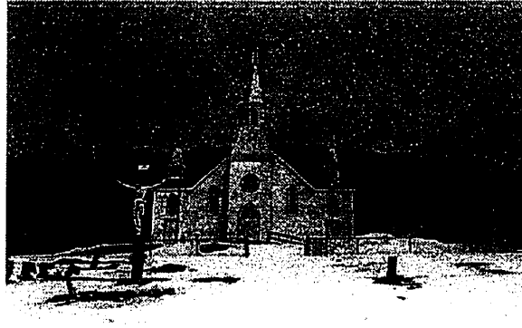
Figure 2.4 Church, Eskasoni, NS
