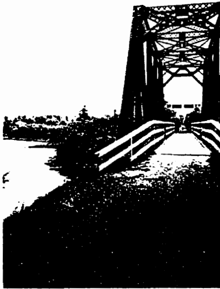
Figure 2. Steel Truss Bridge on Musquodobit Harbour Rail-Trail Source: T.Baker
