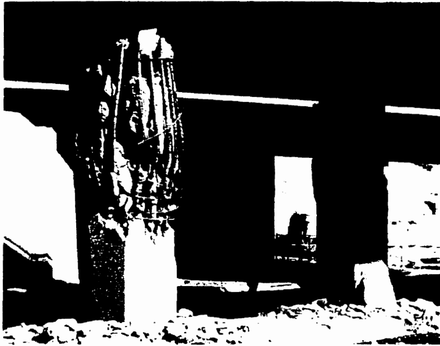
Figure 1.1 Columns of Bull Creek Channel Overpass at Hwy. 118 damaged during the 1994 Northridge Earthquake. (Saatcioglu, 1994)
