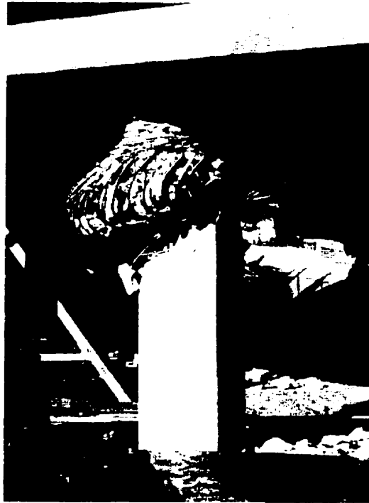
Figure 1.3 Column shear failure of Bull Creek Channel Overpass at Hwy. 118 damaged during the 1994 Northridge Earthquake. (Saatcioglu, 1994)
