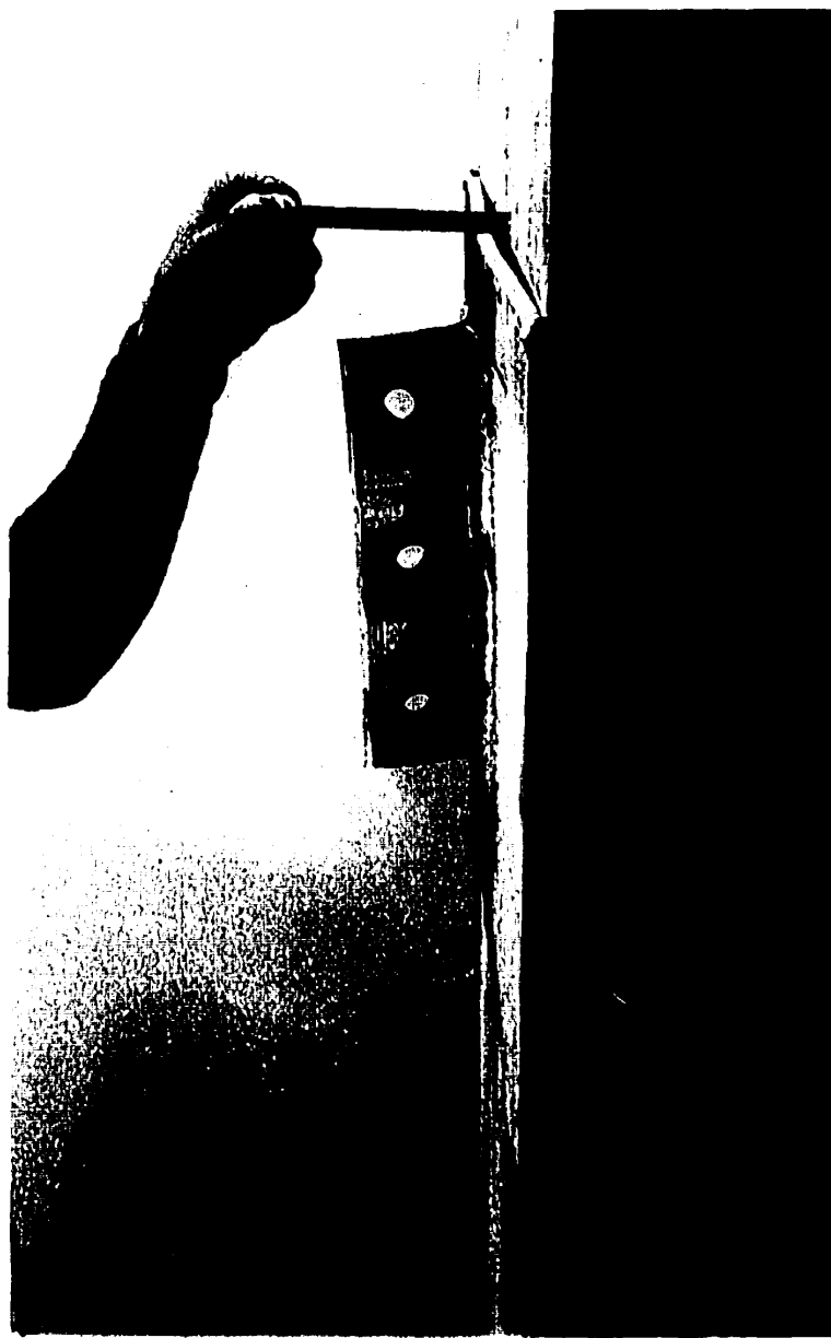
Figure 4.17: View of Failed Specimen C600-W410-LDA-C
